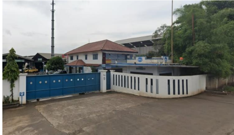
Gambar 3.2 : PT. Duta Hita Jaya Plant Setu
